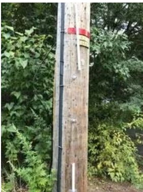
A vandalized PVC pipe, marking an eruv, on Airmont Avenue in Mahwah. (Photo: Tom Nobile/NorthJersey.com file photo)
