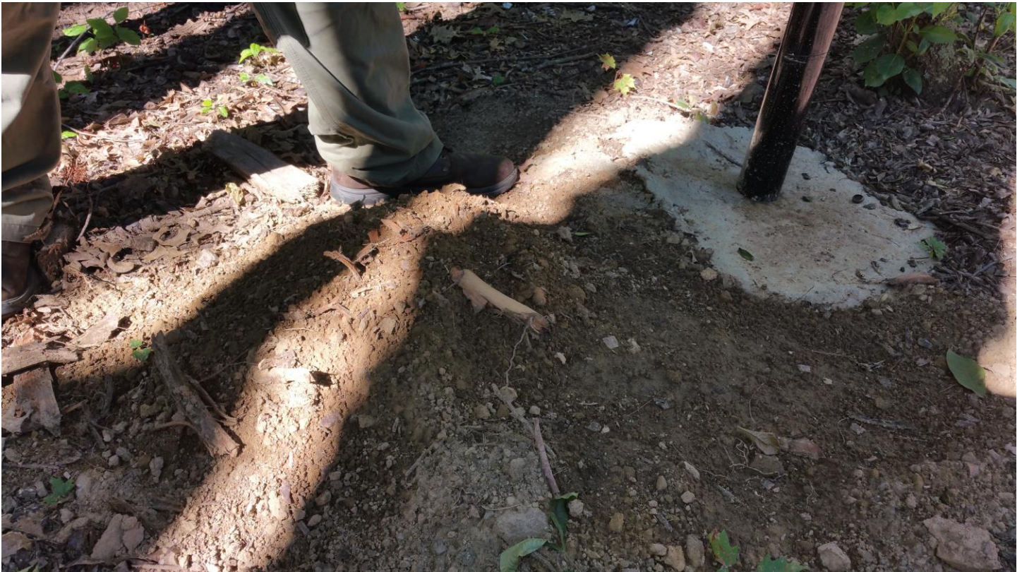
Excated soil should have been removed not just left as a pile of dirt. Cement should have been covered as well.
